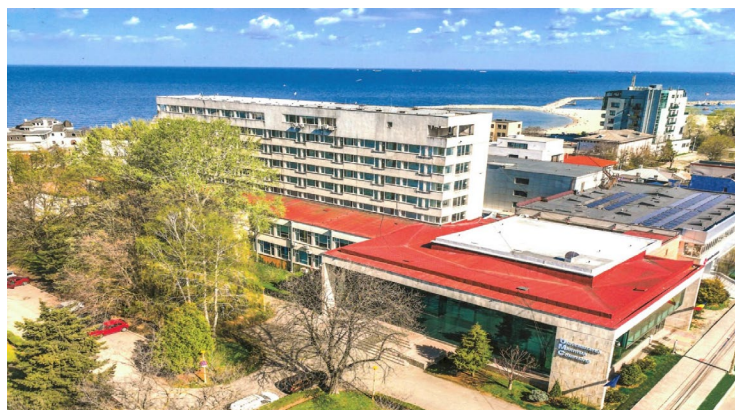
Constanța Maritime University (city center) Mircea cel Bătrân Street no. 104, Constanța 900663, Romania
